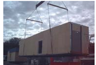
Set the sections on the slab
