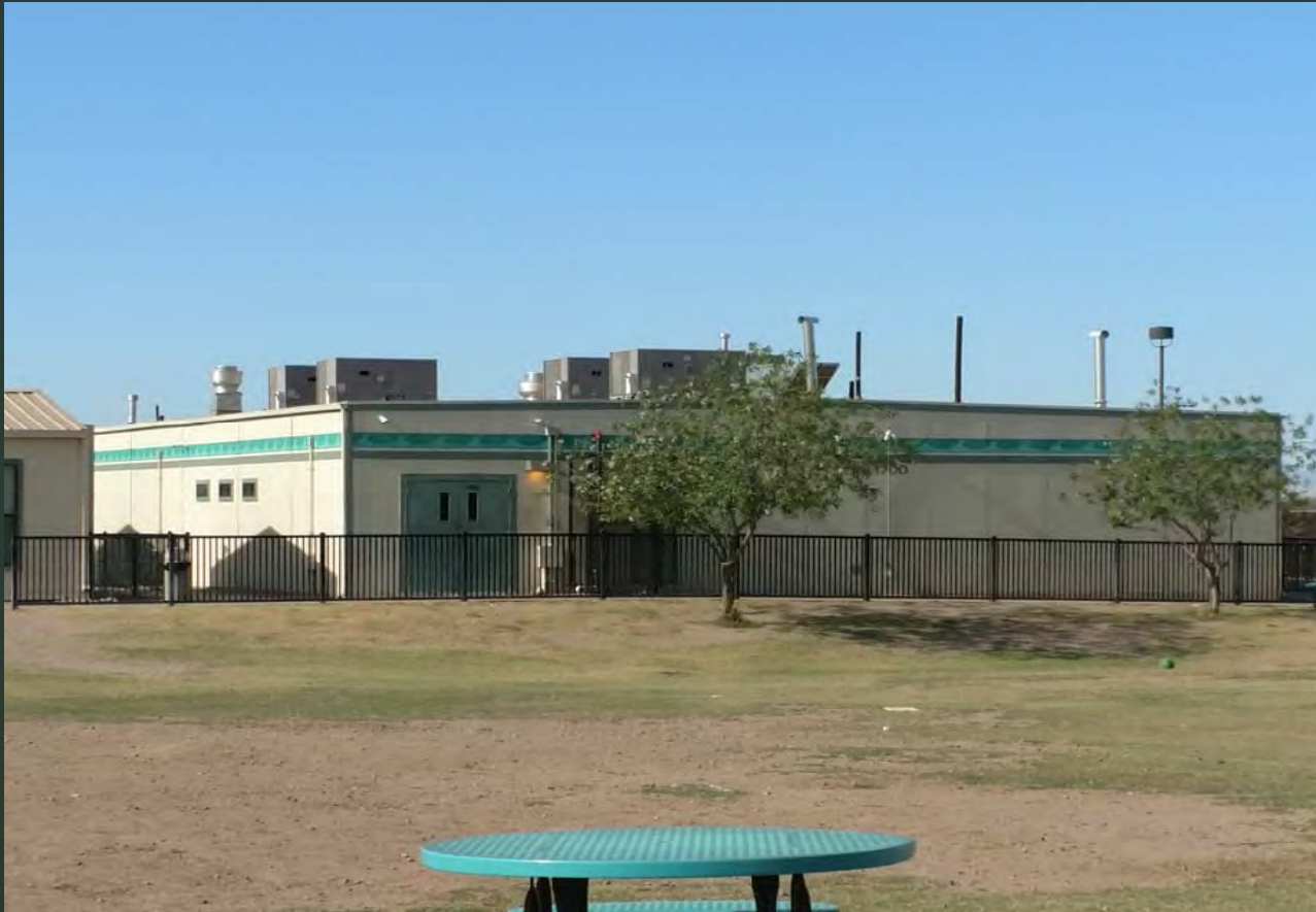
BLACKWATER COMMUNITY SCHOOL- COOLIDGE, AZ
