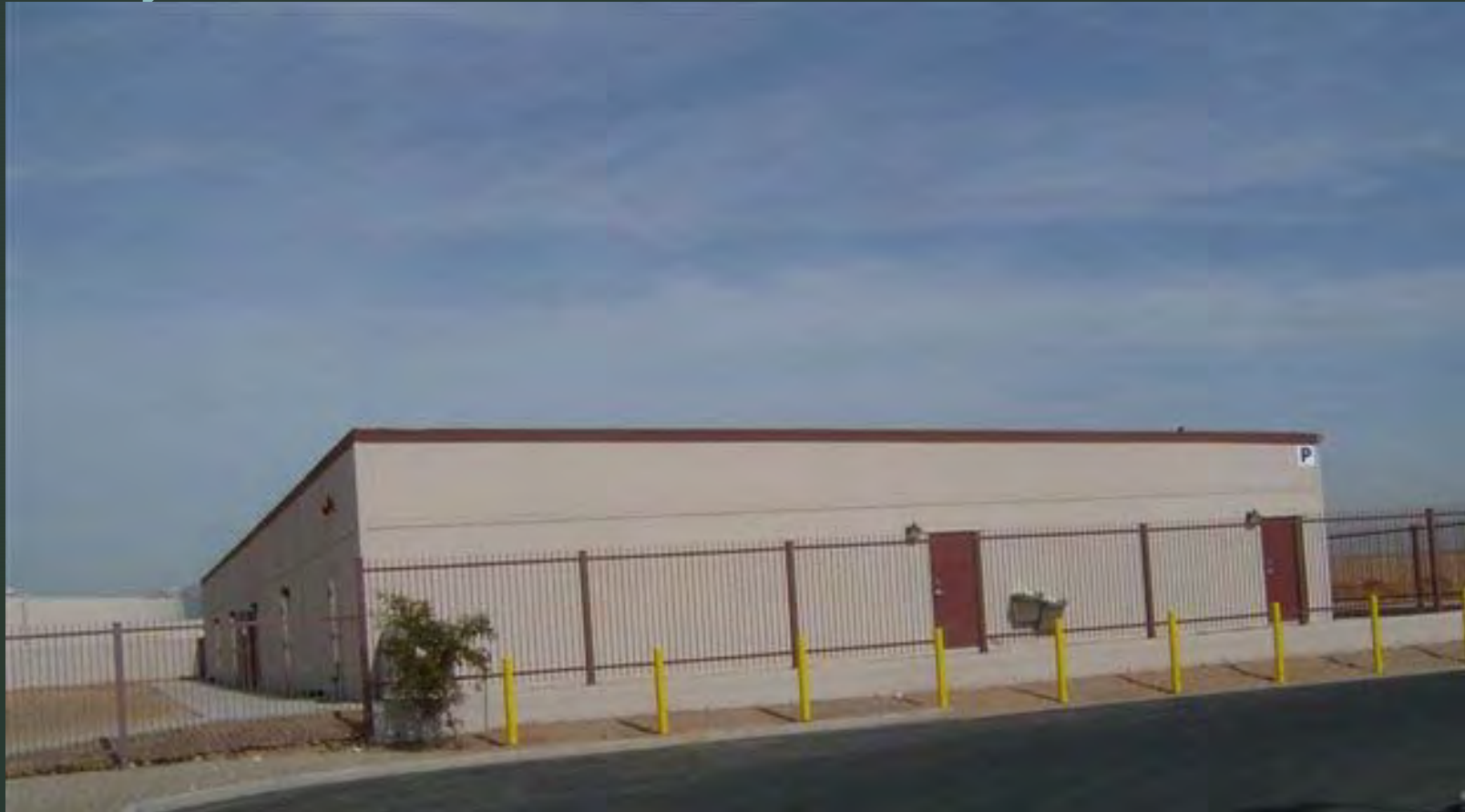
BALES ELEMENTARY SCHOOL – BUCKEYE, AZ
