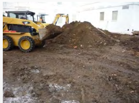
Grading, Pad Preparation
